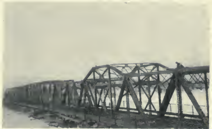
New Steel Bridge completed March 9th.
